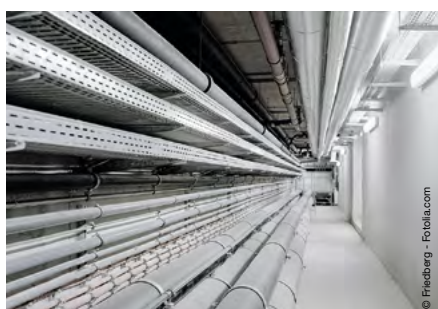
Fixing of cable ducts
