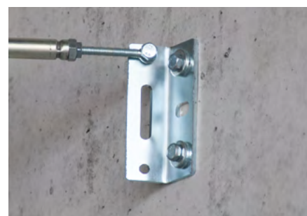
Fixing of brackets and console bearers
